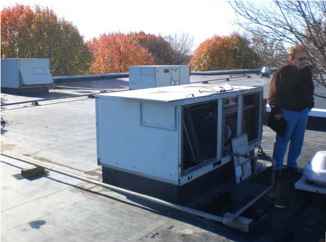
Figure 1. Photo of the roof of test building during installation of controls and test equipment
